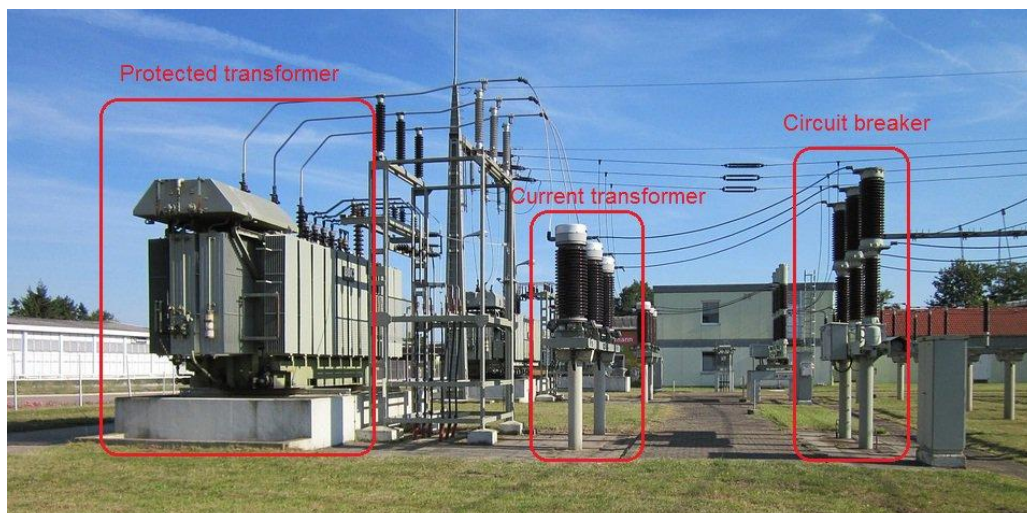
Figure 4. Transformer station
