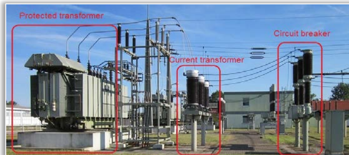
Figure 4. Transformer station
